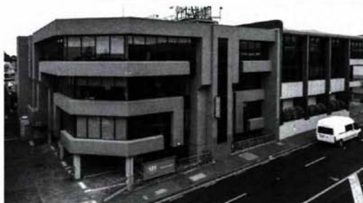
SOLD at $7.45 million - office property at 131 Khyber Pass Rd, Auckland
