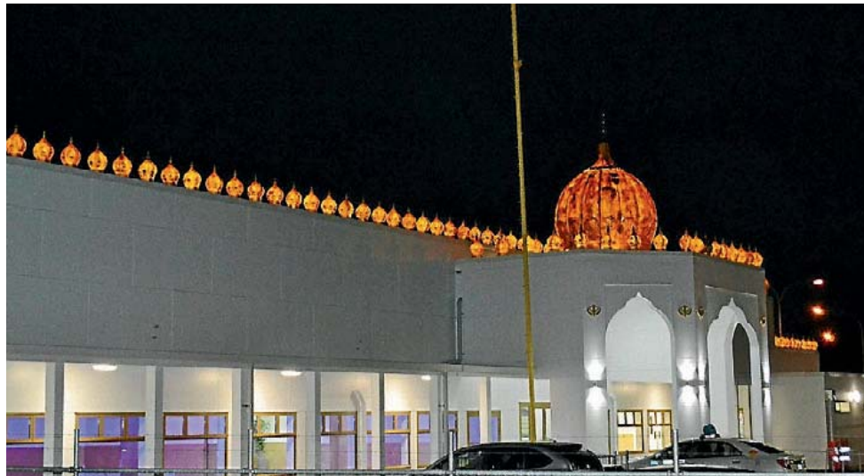
The Sikh temple in Naenae, transformed from a supermarket building by Arc Design's Ananth Sharma.
