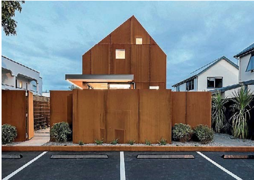
Rusted Corten steel features on the exterior of the Madras Street units in Christchurch designed by Mitchell Coll of Coll Architecture.
