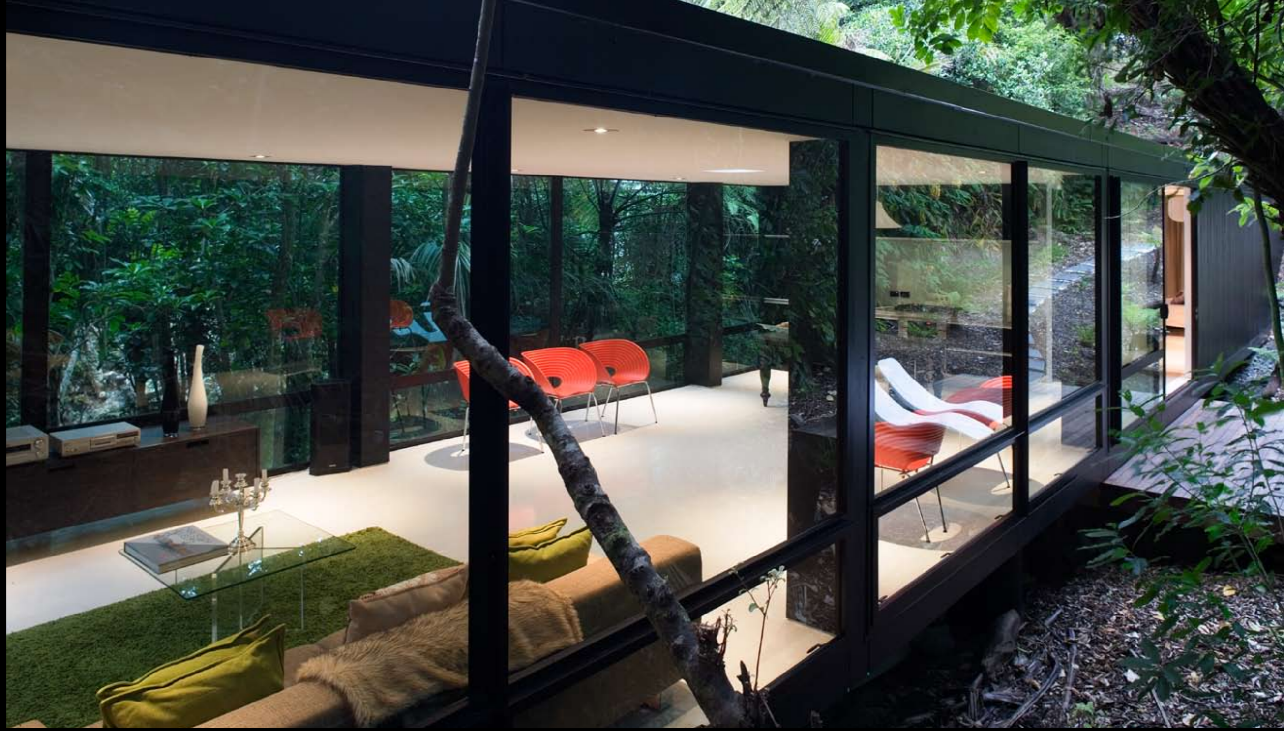
Special flat beads were applied to fixed lights above opening sashes to ensure continuous sight lines
