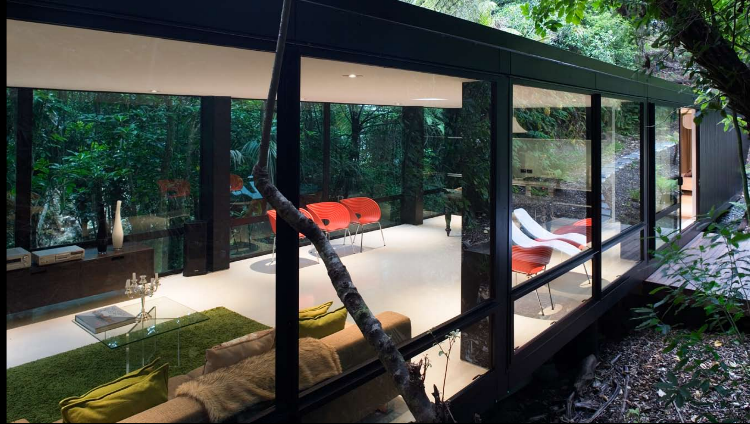
Special flat beads were applied to fixed lights above opening sashes to ensure continuous sight lines
