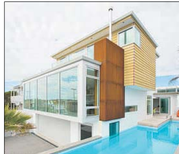
WINNING DESIGN: A four-bedroom, three-level beach haven in Papamoa Beach Rd.
