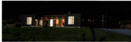
Residential New Home between 150sqm and 300 sqm Potter Hart House (Wellington) designed by Brynna McCauley of BMC Design Ltd Judges' comments: The house sits beautifully on its site, uncompromised by fussiness around any of its edges.
