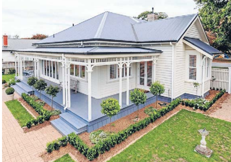
The villa posed numerous challenges for Waikato architectural designer Aaron Guerin such as relocating the original home and a protected tree on site.
